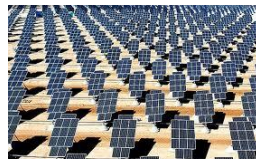
Solar Power plants
