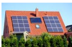
On-grid residential roof-tops
