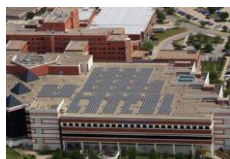
On-grid commercial/ industrial roof-tops
